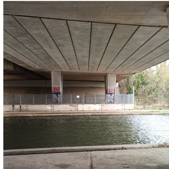
Figure 2: View of underside of eastern deck showing joints
