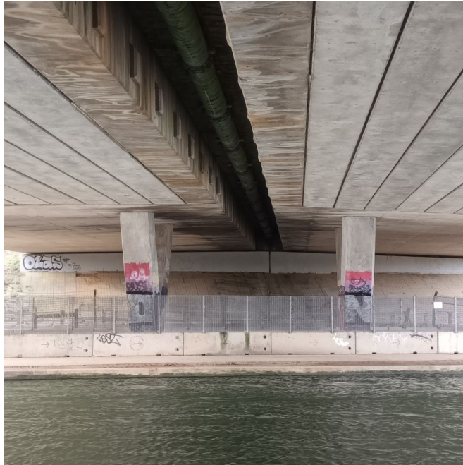
Figure 3: View of central reservation from below showing pipework
