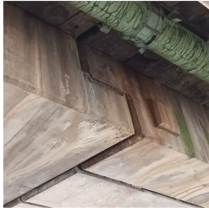
Figure 4: View of western reservation showing expansion joint and additional longitudinal joints
